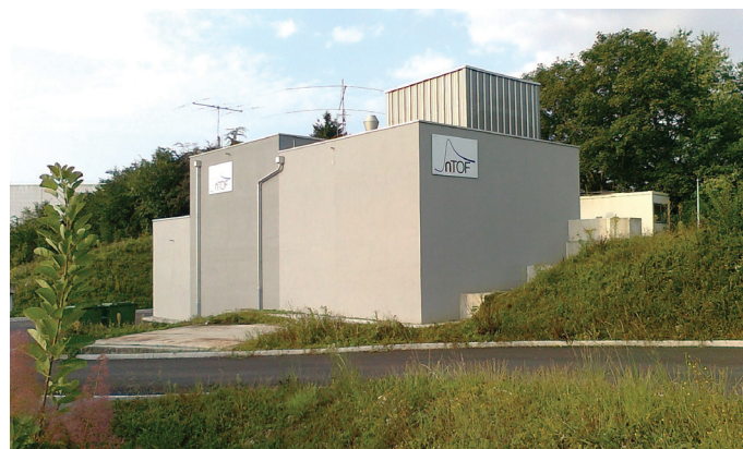
The new EAR2 building for the n_TOF neutron source. (OPEN-PHO-CIVIL-2015-002 – 1)
