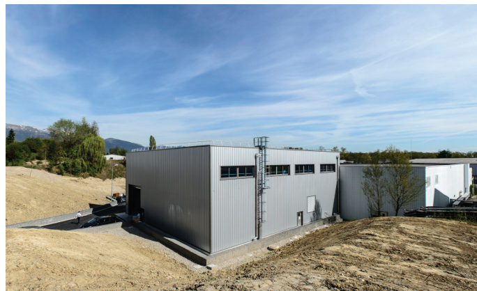
The new ELENA building was inaugurated after less than a year's construction work. Some 10 000 tonnes of earth had to be moved by around 500 lorries. (CERN-PHOTO-201404-075 – 1)
