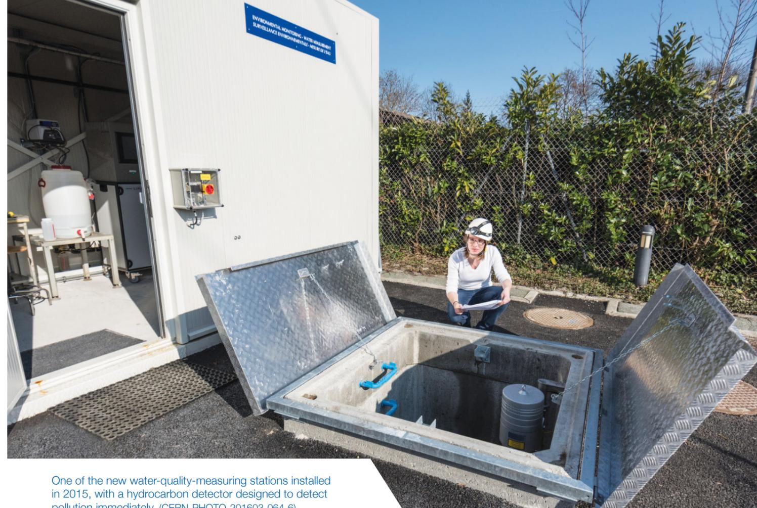
One of the new water-quality-measuring stations installed in 2015, with a hydrocarbon detector designed to detect pollution immediately. (CERN-PHOTO-201603-064-6)
