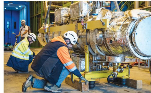
Preparation of one of the new beam absorbers for injection, installed during the year-end technical stop. (CERN-PHOTO-201601-004-8)
