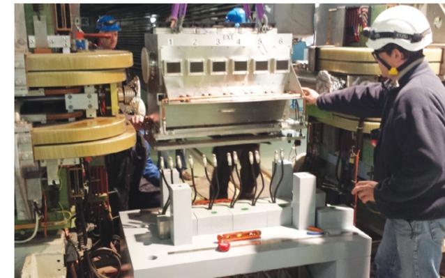
Installation of a FineMet cavity in the PS accelerator for the stabilisation of high-intensity beams. (OPEN-PHO-ACCEL-2016-003-5)
