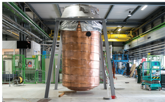
A new cryostat for testing future superconducting cables is being installed in the SM18 test hall. (CERN-PHOTO-201603-062-1)
