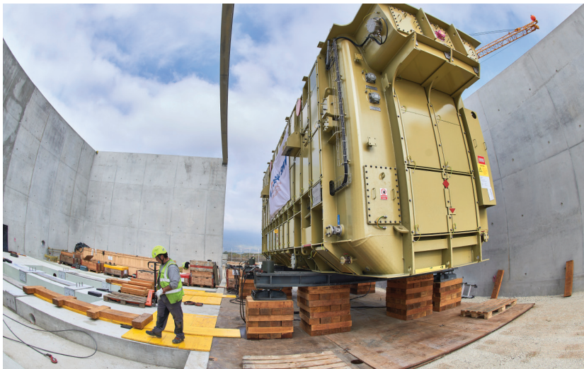
A new 400 kV power transformer, the largest at CERN, was delivered to reinforce the Laboratory's electrical infrastructure. (CERN-PHOTO-201810-254-31)
