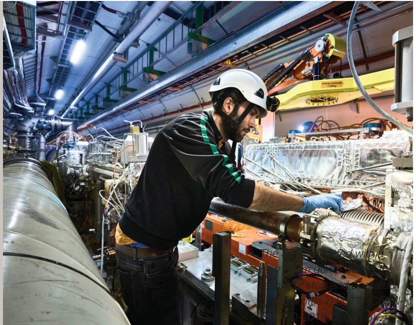
New collimators developed for the High-Luminosity LHC were installed in the LHC, two of them near the ATLAS experiment. (CERN-PHOTO-201801-011-1)
