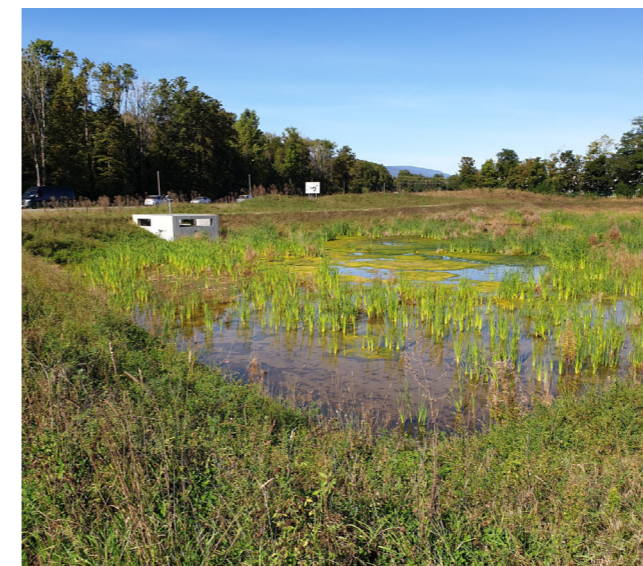
Retention basin that receives rainwater from the CERN Prévessin site, allowing the regulation of run-off into the Lion and the retention of accidental pollution.
