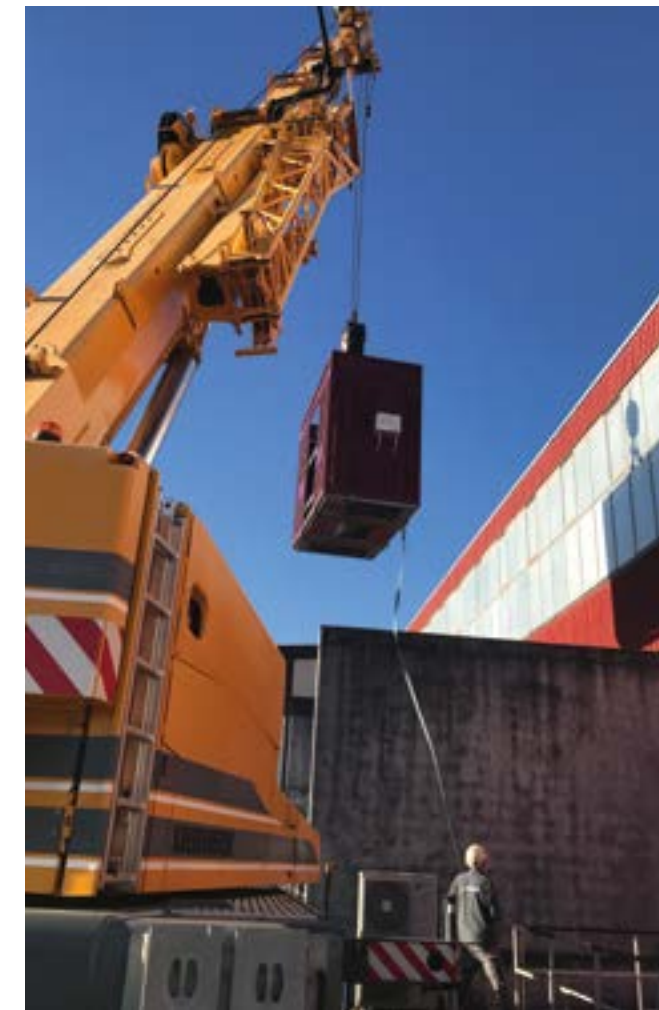
Installation of a dry transformer
