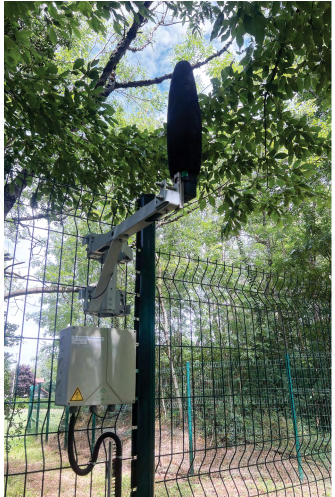
Noise monitoring station at LHC Point 4 (Échenevex, France).
