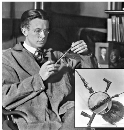
Fig. 4: E.O. Lawrence and his 5-inch cyclotron, the first successful cyclotron built by Lawrence and his graduate student M. Stanley Livingston, (Credit: Lawrence Berkeley National Laboratory).
