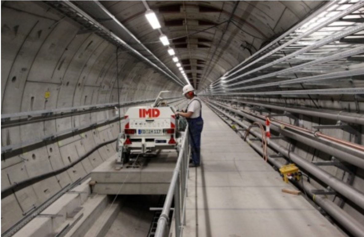
Fig. 7: The empty XTL tunnel at DESY Hamburg with the lights as the only heat sources
