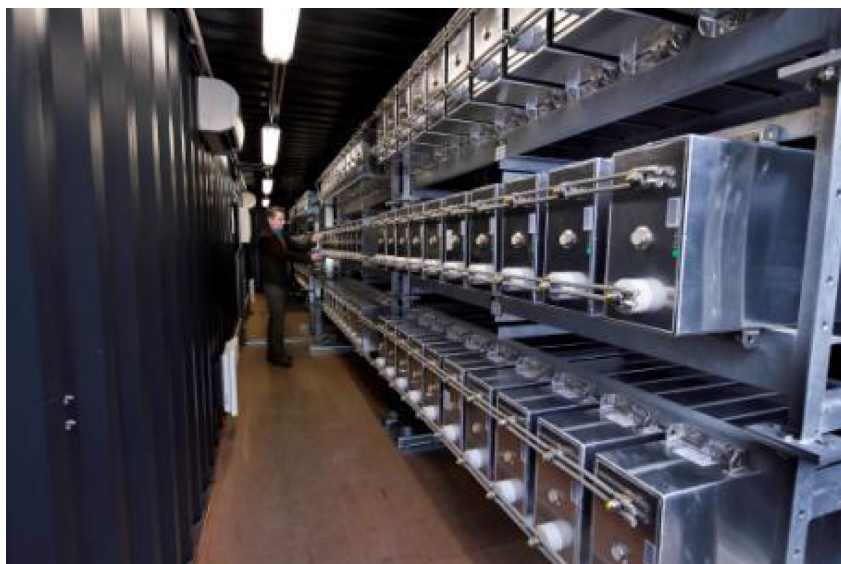
Fig. 22: Photo of one of the six DC storage capacitor banks inside its container
