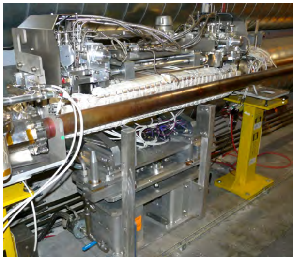
Fig. 31: Active absorber TCLA.B6R7.B1 as installed in the betatron cleaning insert. The stepping motors that control jaw position and angle are visible on top of the vacuum tank. The pipe of the opposing beam is also shown.
