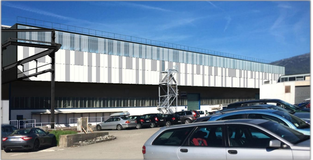
Fig. 5-8: Architects 3D rendering of future upper Northeast façade.
