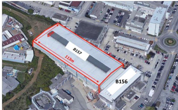
Fig. 5-2: Sky view of Buildings 157 and 156.
