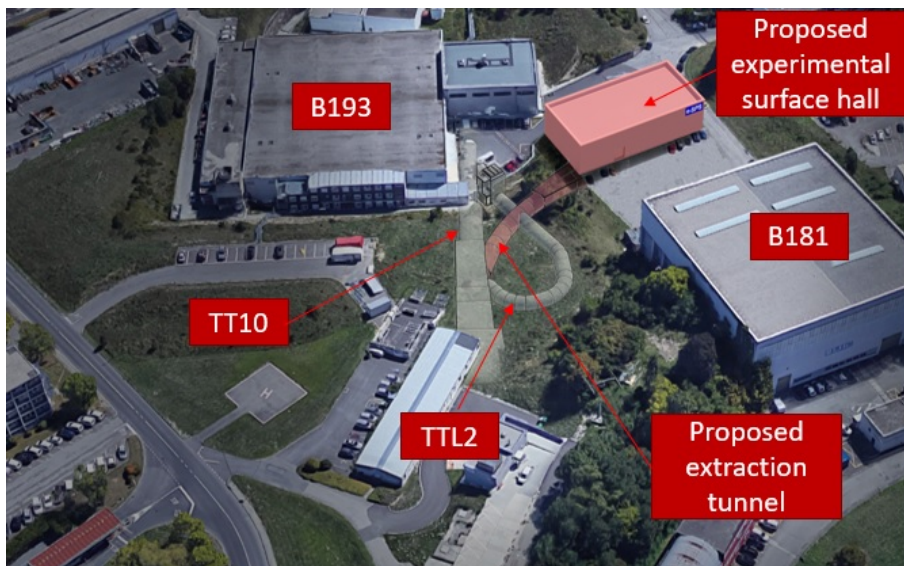
Figure 5.65: Birdseye visualisation of the proposed facilities in red showing surface and buried structures.
