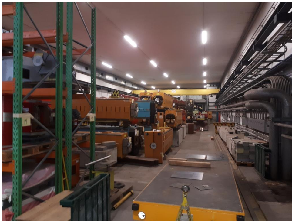
Figure 5.8: View within existing TT5 tunnel looking east towards TT4.
