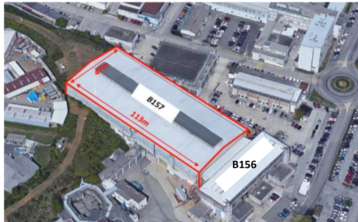
Fig. 5-2: Sky view of Buildings 157 and 156.
