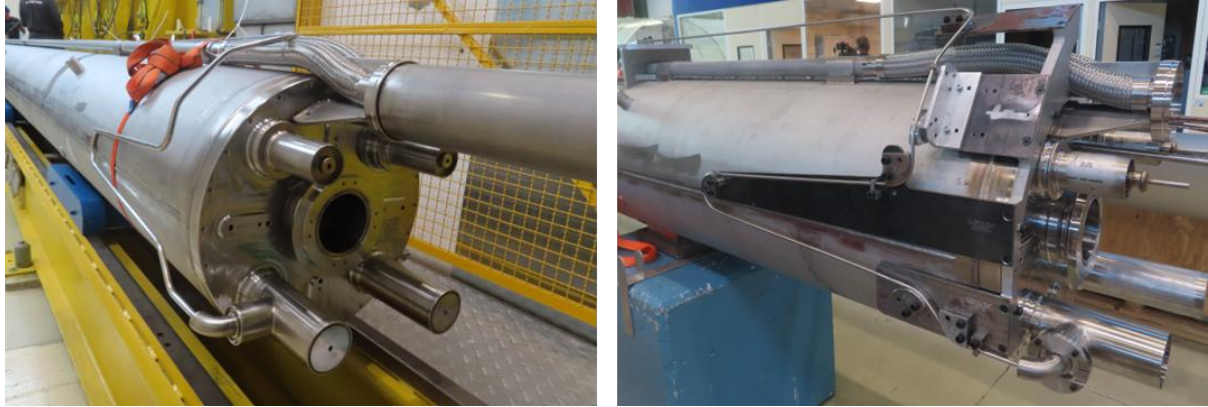
Figure 39: Examples of capillaries used in the assembly of 7.2-m-long HL-LHC MQXF quadrupole magnets at CERN. Left: capillaries installation on cold mass. Right: capillaries installation on thermal shields during cryostating (Courtesy of O. Housiaux, SERCO, H. Prin and D. Duarte Ramos, CERN).
