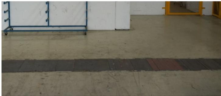
**Fig. 12.8:** Photograph of a typical service trench with steel covering.
