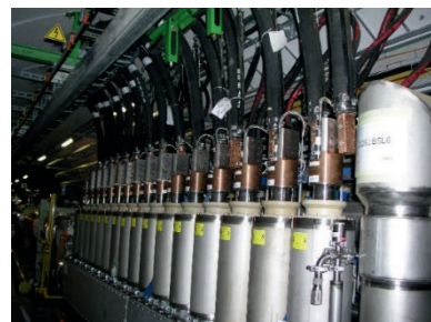
Figure 17-25 – Water cooled cable technology and Water cooled cables used in LHC.
