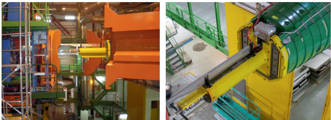
Figure 8-18: Photos showing the CMS forward shielding during access. The small rotating shielding is open showing the yellow beam pipe support module. Details of the beam pipe support and the cable tray to be modified are shown on the left.
