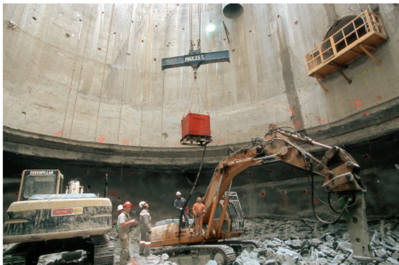
Figure 17-11: Hydraulic hammer method of excavation.
