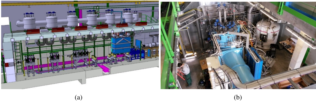
Fig. 9.4: The cryogenics distribution system (a) and the cold box housed in the new building next to the ISOLDE experimental hall (b).
