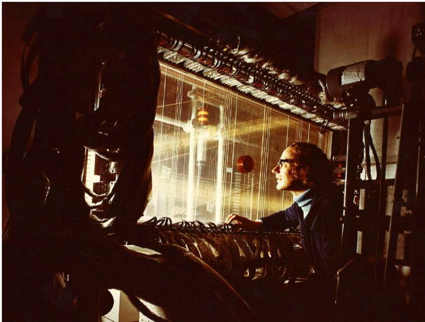
**Fig. 6:** The picture shows Roger Clift working on one of the proportional chambers which were situated within the Forward Spectrometer magnet P1, P2, P3. The central brown region is the desensitized area through which the muon beam passed (image credit CERN, photo X-611-9-77).
