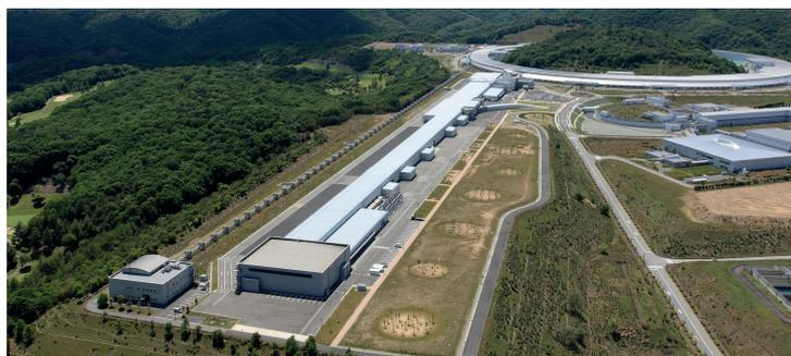
**Fig. 75:** SACLA FEL top view from <http://xfel.riken.jp/eng/>. In the long building is installed SACLA with the different FEL branches, whereas in the rear of the picture, one of the third generation storage ring beamlines, a very intense laser, and SACLA photon beam can be coupled. The configuration also enables to use the linac electron beam to inject in the storage ring for very short pulse synchrotron radiation production.
