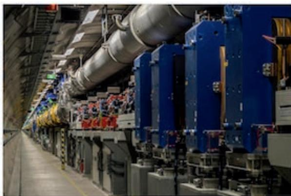
**Fig. 80:** View into the accelerator tunnel: electrons guided into the first four superconducting accelerator modules (yellow) and in a chicane (in front, blue and red), from [531].
