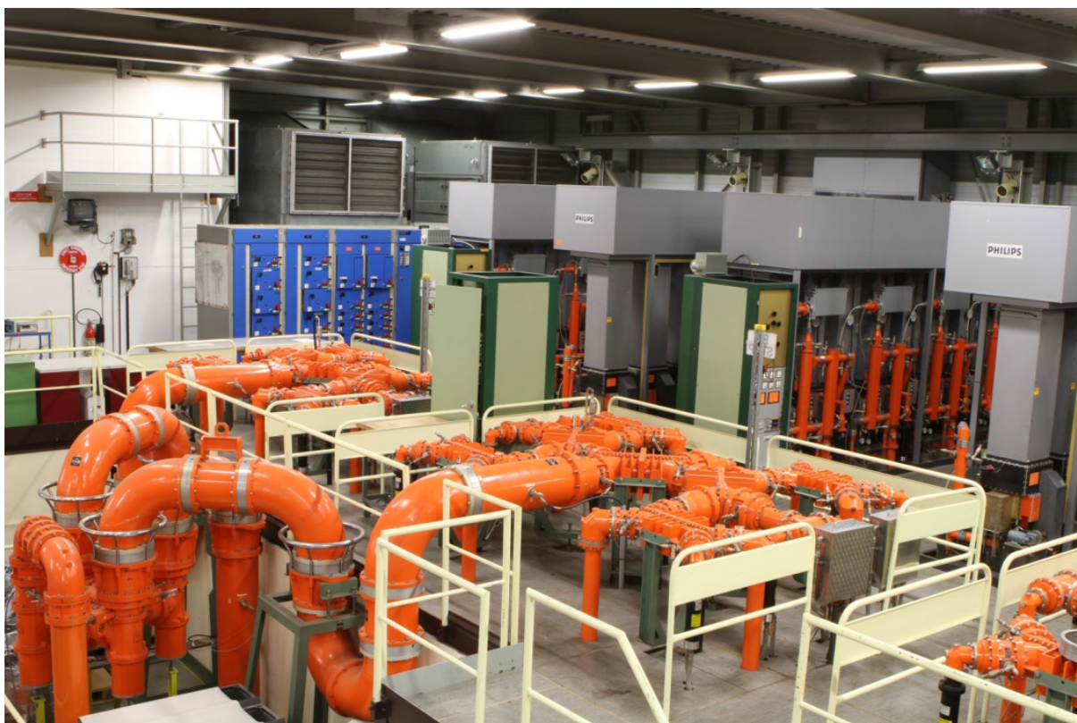
Fig. 36: CERN SPS 64 to 1 combiner @ 200 MHz
