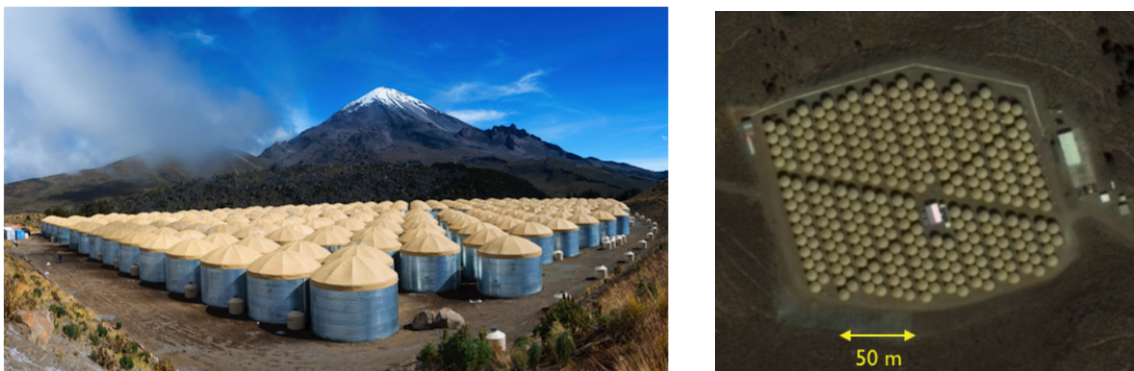
Fig. 11: Views of the HAWC array of water tanks. Left: ground view (J. Goodman, 2016). Right: satellite view; at the centre is the Counting House with the electronics and computing; on the right is the HAWC Utility Building with the water filtration plant (Google Earth, 2016).
