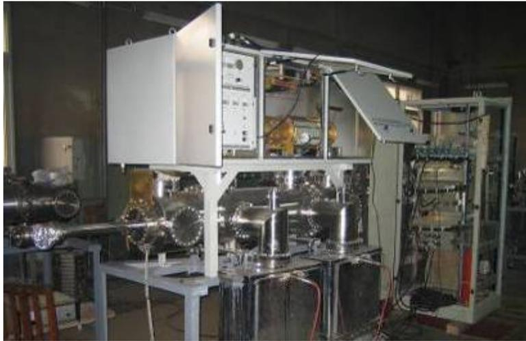
**Figure 5:** A kicker installed in the BEPCII tunnel
