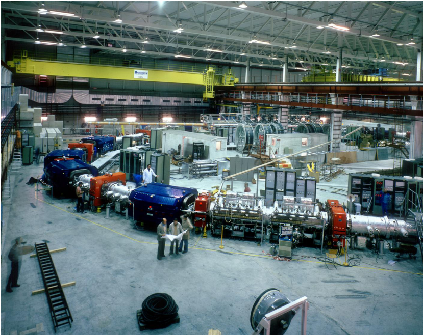
Fig. 2. View of the Antiproton Accumulator during construction.
